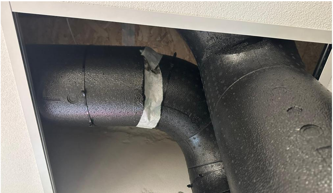
Figure 2 - Air leakage
