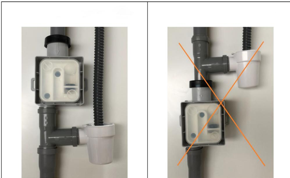
Figure 4 - Correct and incorrect condensate drain connection
